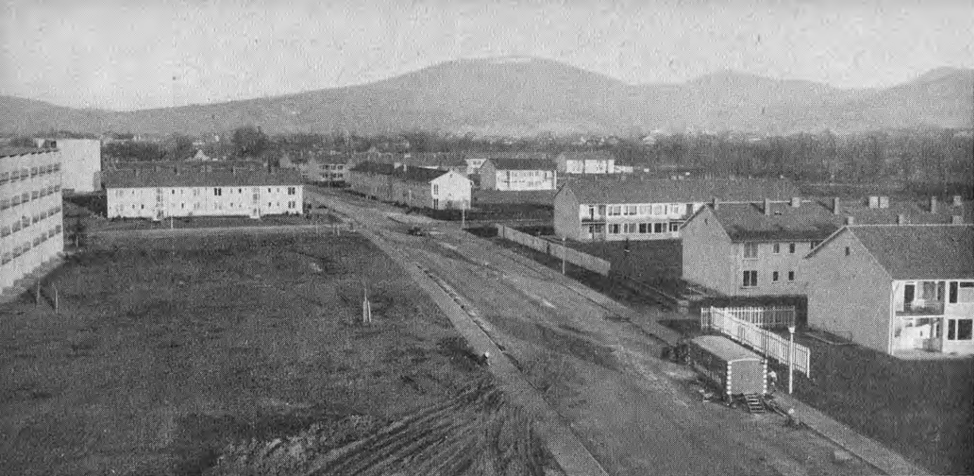
Transfer from Frankfurt of more than 600 German employees and their dependents to reinforce the German staff stationed in Bonn, necessitated the provision of adequate housing accommodation and to that end two large settlements were built on conveniently-located sites not far from HICOG's new headquarters. Pictured above is the "Riepalsche Wiese" project.
