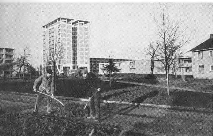
View of the big new Muffendorfer project shows the 10-story structure, one of the tallest in the country, built to accommodate bachelors of HICOG's German personnel.
