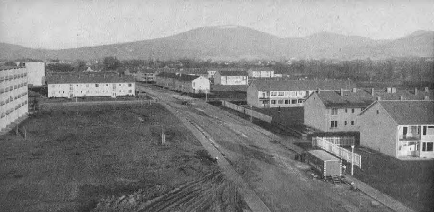
Transfer from Frankfurt of more than 600 German employees and their dependents to reinforce the German staff stationed in Bonn, necessitated the provision of adequate housing accommodation and to that end two large settlements were built on conveniently-located sites not far from HICOG's new headquarters. Pictured above is the "Riepalsche Wiese" project.
